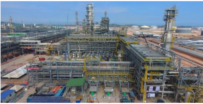
Malaysia, Oil refinery
