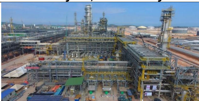
Malaysia, Oil refinery
